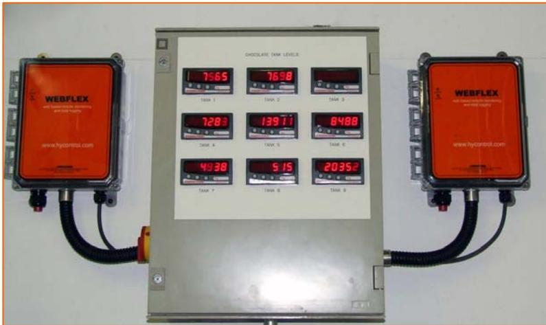
The Webflex system provides a number of key operational benefits and, because it runs on standard Internet Explorer, does not require any specialist software or expensive licenses. Each Webflex unit can take up to six 4-20 mA analogue inputs and six digital inputs. For Bendicks
