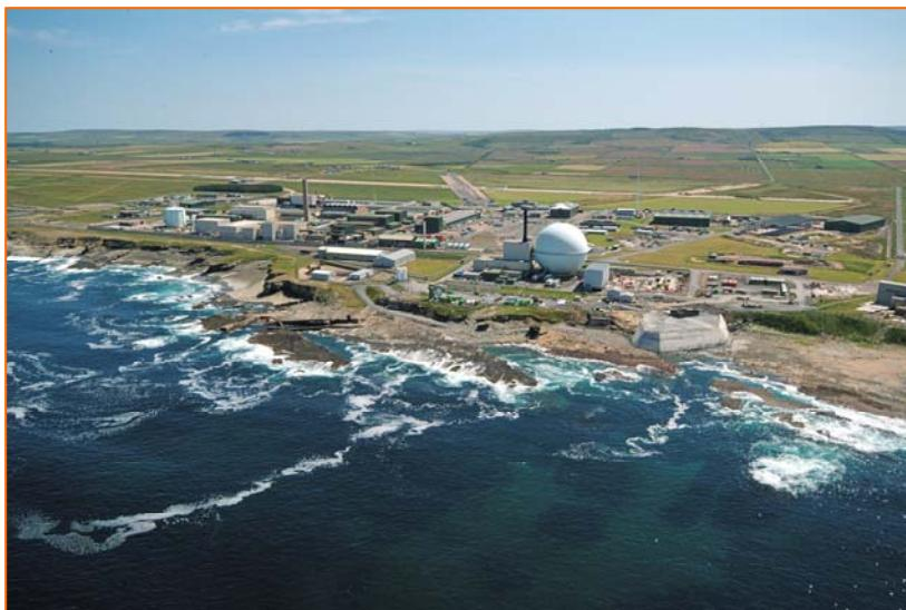
nuclear decommissioning tasks in the world and the site's history in fast reactor and fuel cycle development presents significant decommissioning challenges. Key projects include dealing with liquid metal coolants from the Dounreay Fast Reactor (DFR) and Prototype Fast Reactor (PFR) and managing liquid and solid radioactive waste. It is estimated the clean-up will
