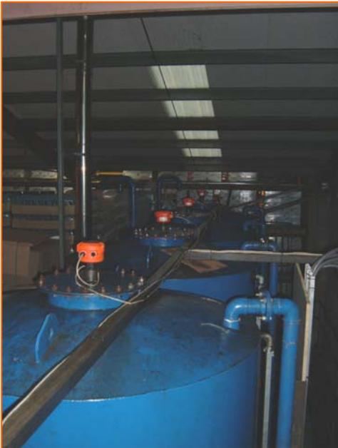
All the level transmitters are powered directly by the WebFlex units which are configured as one master and six slaves. This greatly simplifies the installation and each WebFlex unit can power up to six transmitters, whilst providing the Ethernet connectivity to Maxol's local area network. The master unit is fitted with a GPRS (General Packet Radio Service) modem and this allows highly secure, yet simple to use, access via any standard web browser.
