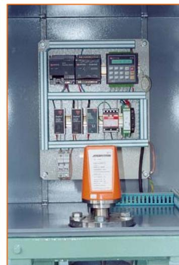
minutes. The unit sends data back to the PLC, 200 metres away in the control room, providing ENDESA with accurate, reliable and maintenance-free level control information. The unit has now been working faultlessly for over four years without any reliability or drift related problems.
